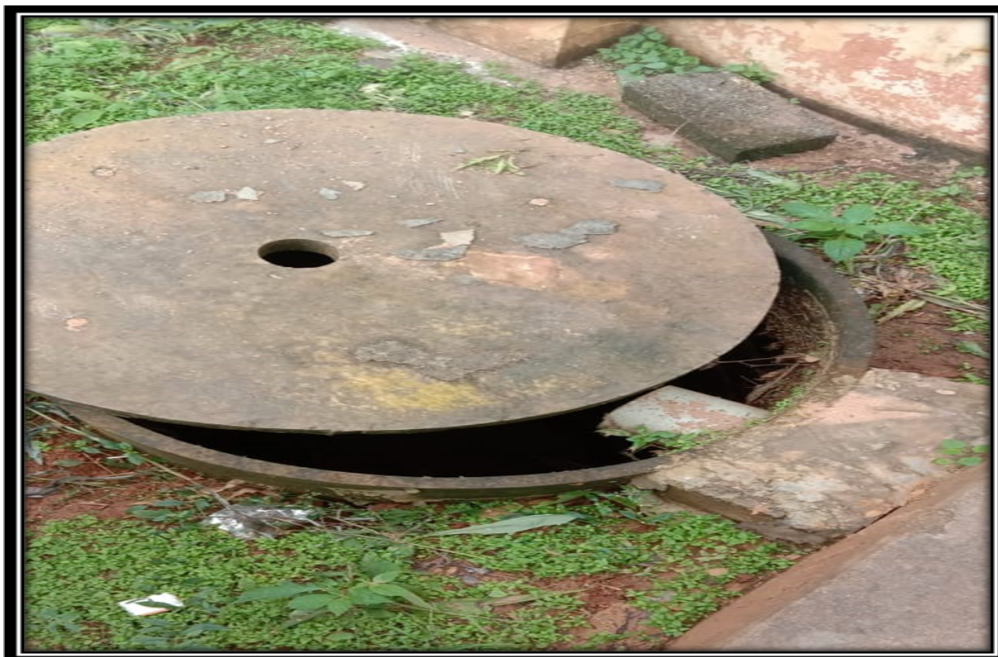
Photo: 11 Rainwater Harvesting
